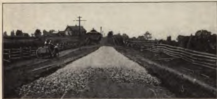
2. Laying the foundation course.
